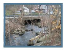
The existing culverts on Southside Avenue and Union Street were in need of replacement. The concrete decks were deteriorating and their integrity was beginning to come into question. This firm designed a culvert replacement solution, prepared the construction documents for the project, and provided management services during the construction phase. This firm was also involved in the coordination with the USACE and the NYSDEC in obtaining the necessary environmental permits for the project.
